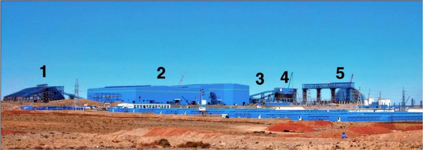
1 - Concentrate storage building. 2 - Concentrator. 3 - Ore conveyors. 4 - Pebble crusher. 5 - Coarse-ore storage building.
